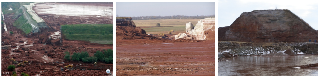
Figure 2 1. Breach of the dam (October 2010); 2. Construction works shown from the inside of the dam (November 2010); 3. Closure of the reservoir with a new, low dyke (December 2010), in the foreground of the cross section of the broken dyke.
